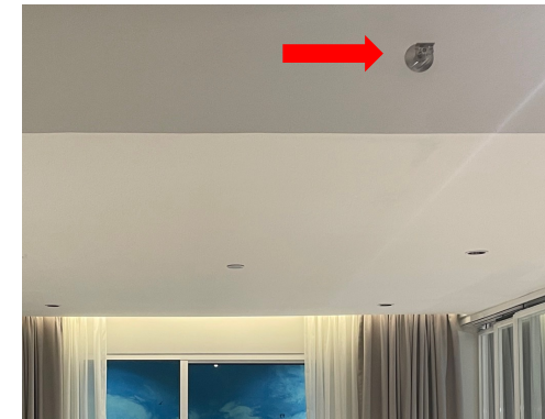
Sidewall sprinkler
